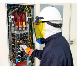
Check electrical installations, loose connections, high resistance in wiring and fuses, overheating of components and corrosion.
